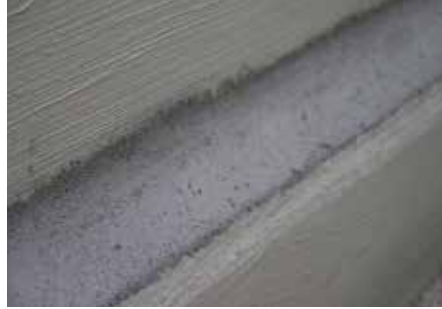
2 Fillet installed with KÖSTER Repair Mortar
