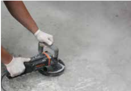
1 Substrate preparation
