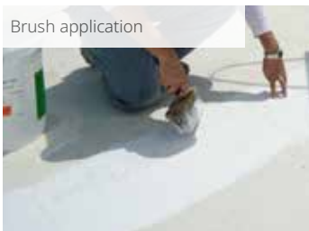
4 KÖSTER Superfleece is applied into the fresh first layer
